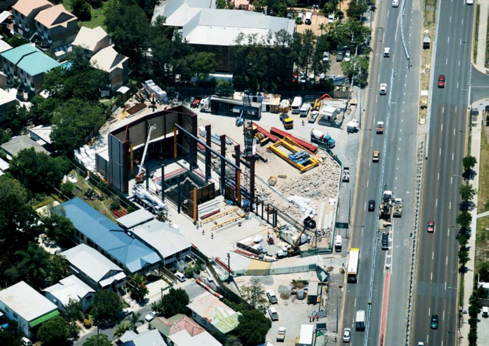
Above: Construction Access Shaft Completed at Shafston Avenue
