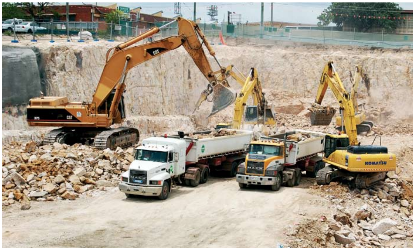
Above: Substantial Construction Progress at Northern Portal
