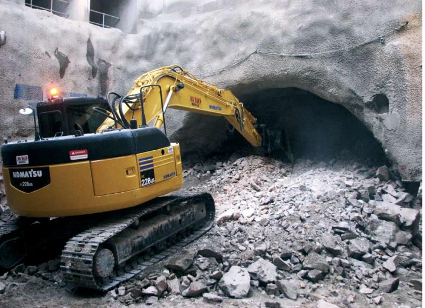
Above: Initial Short Sections of Tunnel at the Shafston Avenue Site
