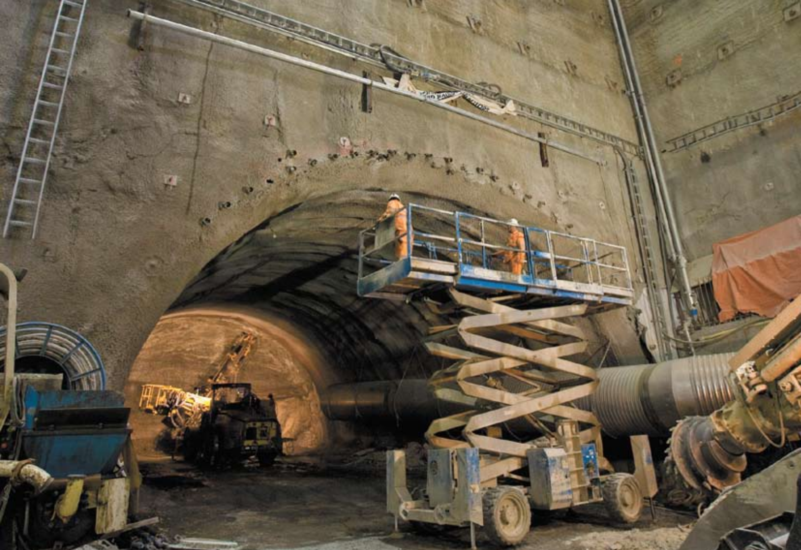
The start of roadheader tunnelling in Woolloongabba.
