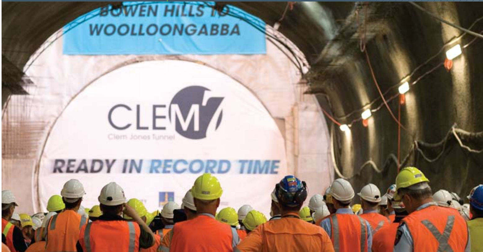
The crew anticipate breakthrough of the tunnel boring machine.
